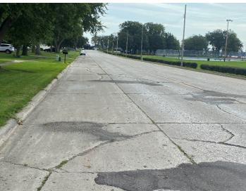
The condition of the existing concrete pavement, curb and gutter, and sidewalk throughout the 8<sup>th</sup> Street NE corridor is poor and pedestrian facilities are largely non-compliant with current ADA standards. As a result, Waseca County is planning for a complete reconstruction of the corridor with new 7.5" thick concrete pavement, concrete curb and gutter, concrete sidewalk, concrete driveway aprons, and pedestrian ramps. Both the City and County are tentatively planning sidewalk
