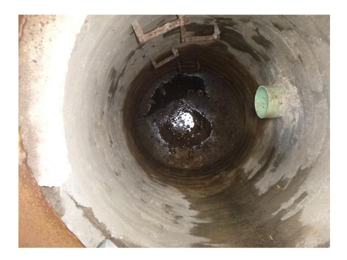
MH 1088 MH Condition – Concrete Block – Fair Ring Condition – Poor Rim Elev. 1132.33 Pipe 8" Clay IE W – 1123.02, Pipe 8" Clay IE S. 1122.0 Inver Poor – 1' inside drop.
