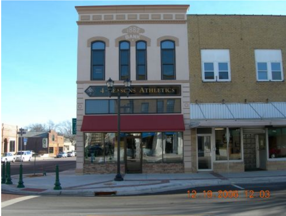
2006 – Four Seasons Athletics – This photo shows a renovated building that has restored the stucco on the front façade. A row of transom windows has been added above the entry door and display windows and now includes a fabric awning. The name of the store has been placed above the transom windows. The windows have also been restored to fill the entire arched opening. “1882 Bank” is still visible at the top of the building.
