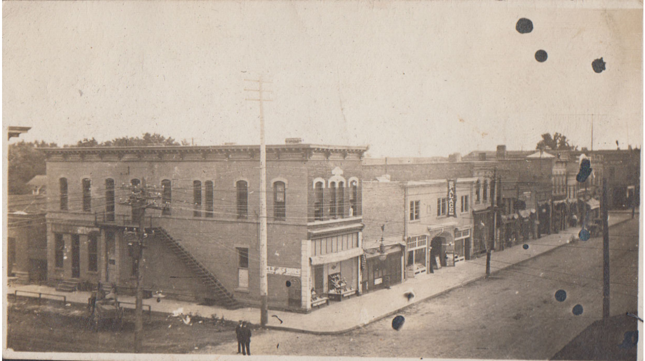
1912 - possibly a shoe store – a store name seems to be painted on the side of the building. Great photo showing the brick façade, iron fire escape, original arched windows, fabric awning, display windows, and recessed entry door.
