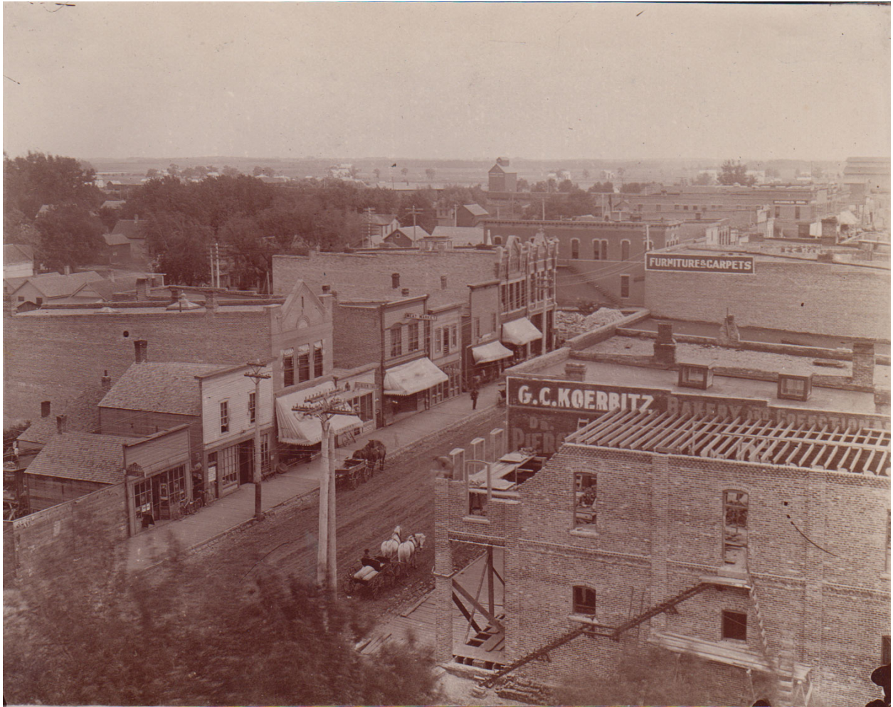
1897 – Bank of Waseca one block down on the left – notice the total brick façade, the arched windows, the Italianate style cornice, and the iron fire escape.
