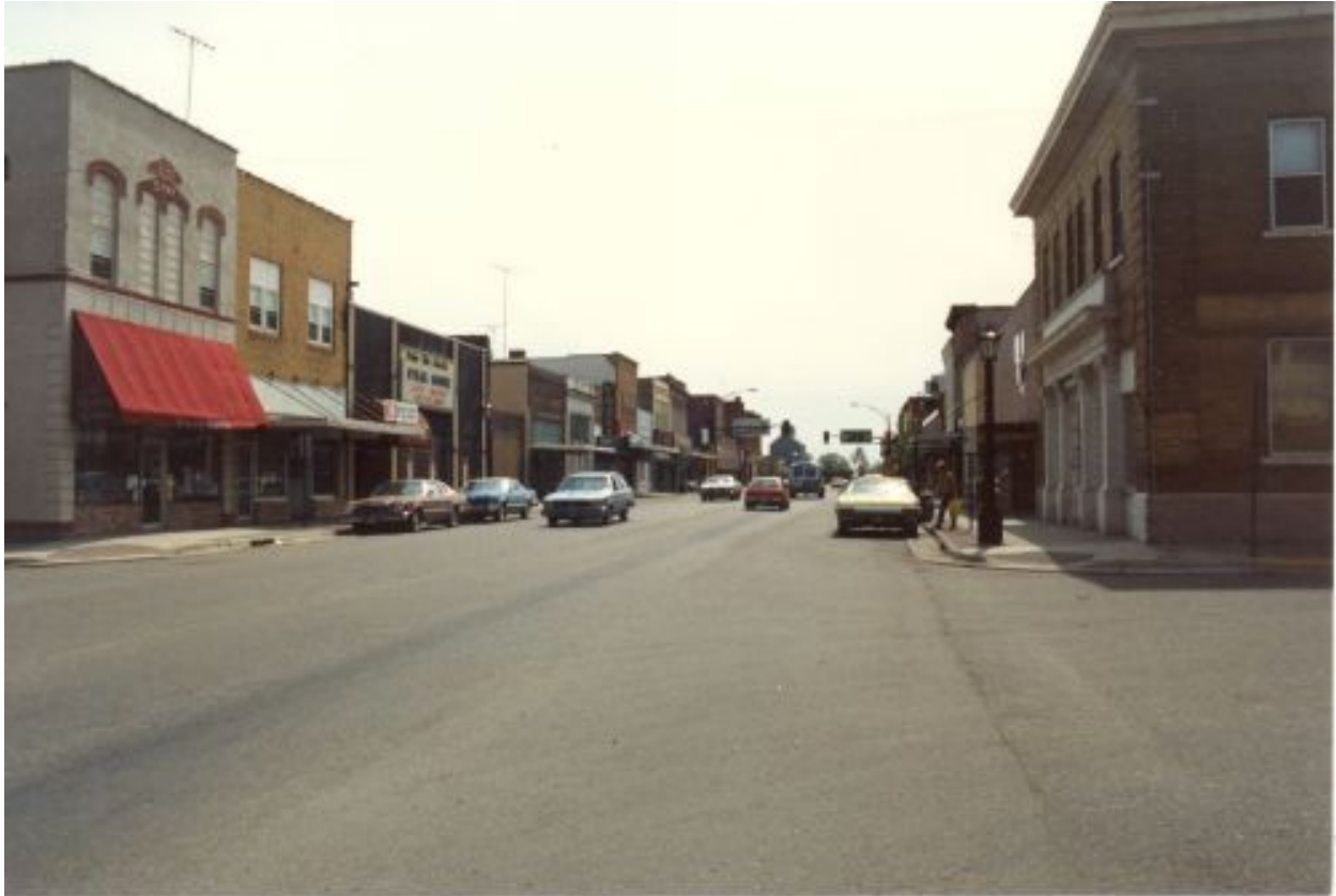
1985 – Four Seasons Athletics on the left with the red awning – Some restoration work has begun on the main façade including the addition of a large fabric awning. Also, the hanging sign has been removed.
