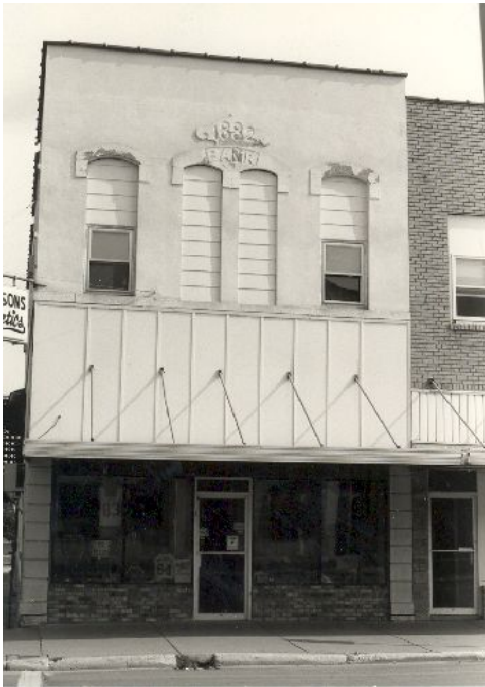
1983 – Four Seasons Athletics – Hanging sign located just to the left of the picture. Stucco has been added to the front façade at some point. Notice the raised stucco plate that reads “1882 Bank” is still present at the top of the building. The original arched window openings are visible, although they are either shuttered or have small replacement windows at this time. The transom windows have been covered.
