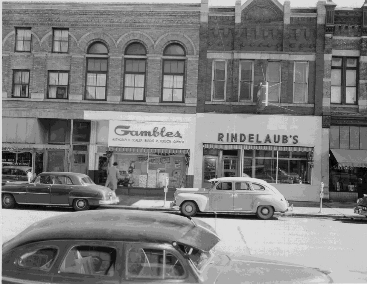
1956 – Waseca Sports Shop occupies 210 State Street North (on the left). A Gambles store occupied the space for 208 State Street North. You can see in this photo at some time in the 1940s, the windows above Waseca Sports Shop were changed and the brick archways were altered.
